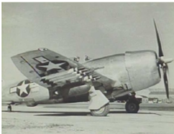
This P-47 THUNDERBOLT demonstrates mission flexibility with its mixed load of bombs, rockets, and .50 caliber machine guns. The ability to provide a variety of weapons effects, when and where needed, was a major part of counterland success in World War II.
